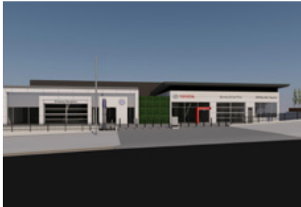
Bill Buckle Service Centre, Brookvale
